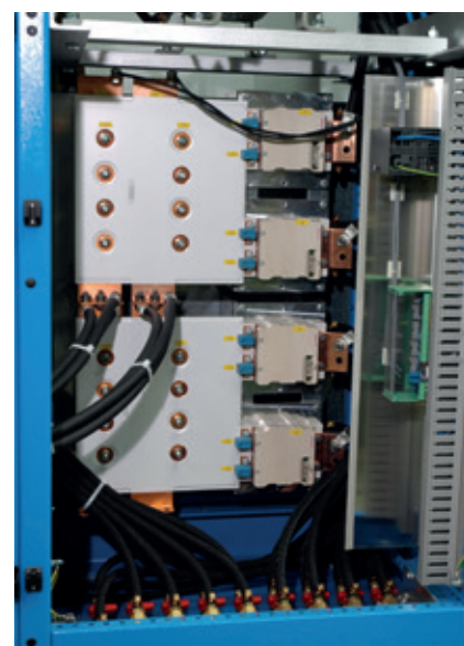
IGBT converter for 3,000 kW
