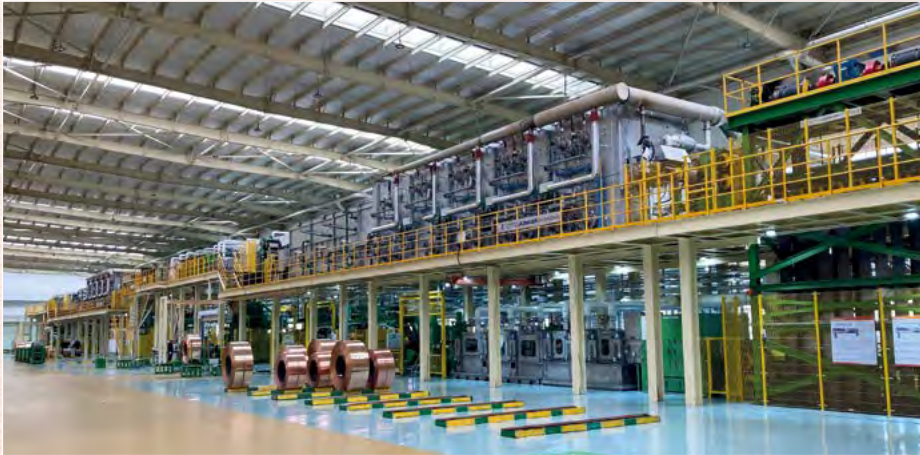
Strip Processing Line, Annealing & Pickling Line with Vertical Annealing Furnace
